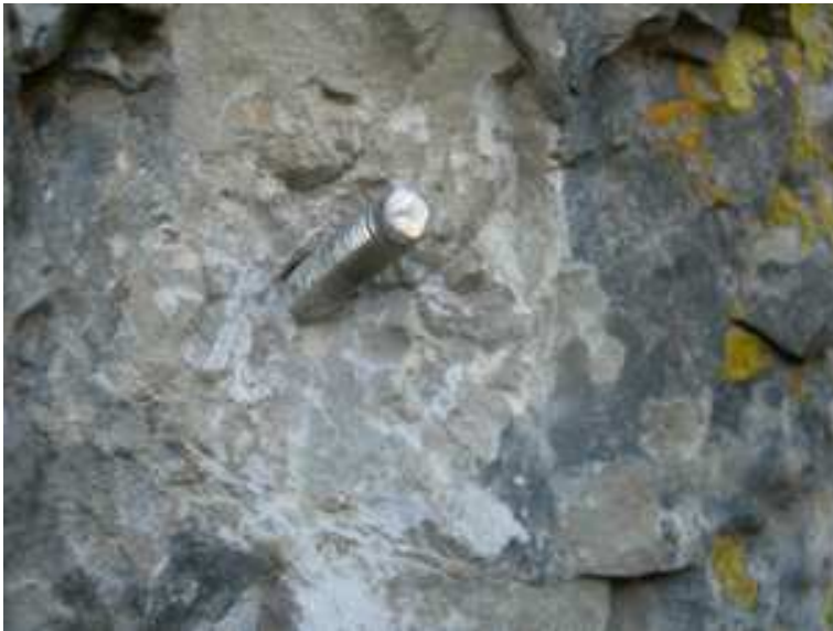
Rock fracture around a bolt
