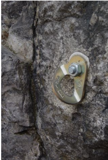
Glue-in threaded bar anchor, with a Fixe hanger.
