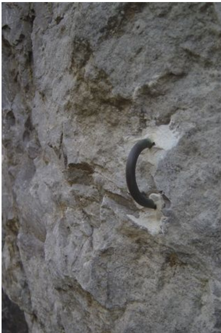
Home made staple anchor.
