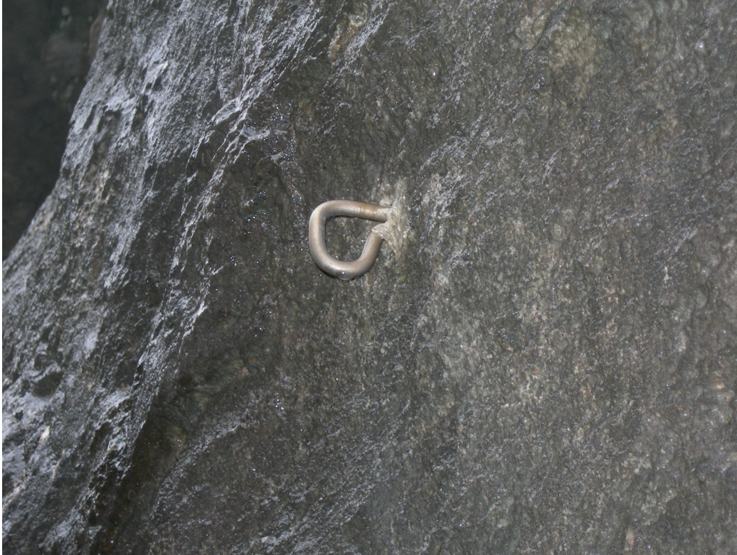
Eco anchor placed in a drainage line
