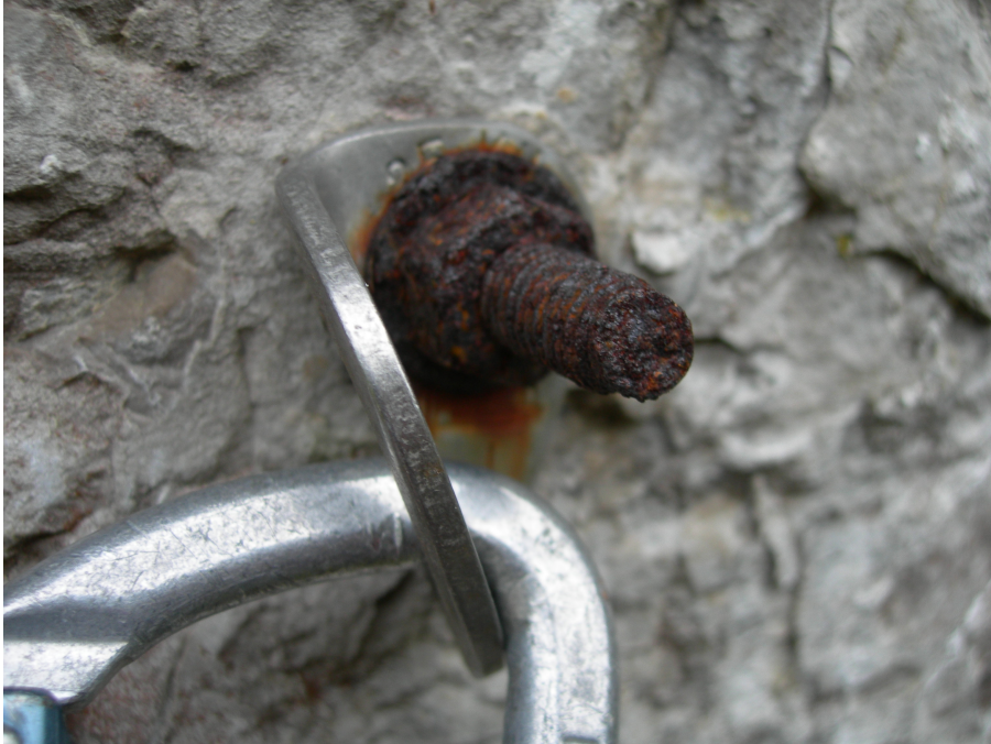
Stainless steel hanger, mild steel bolt
