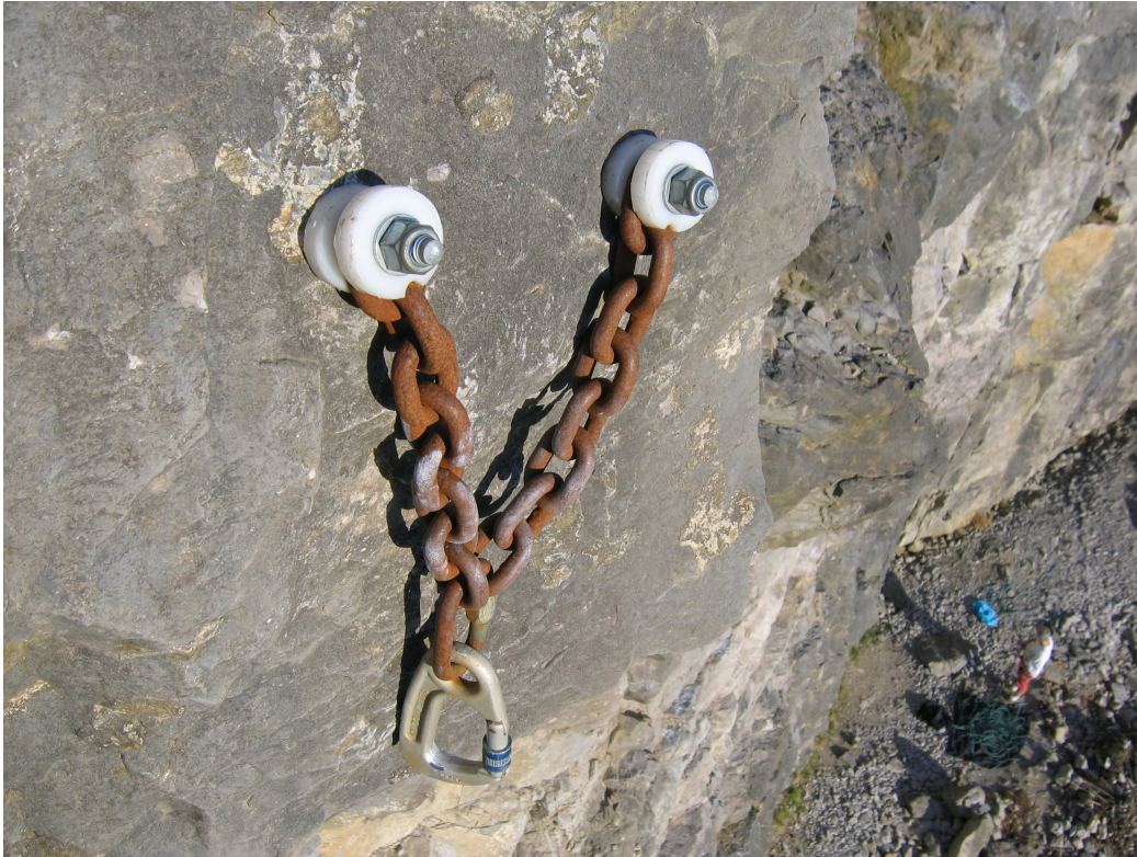
A homemade lower off at Horseshoe Quarry.
