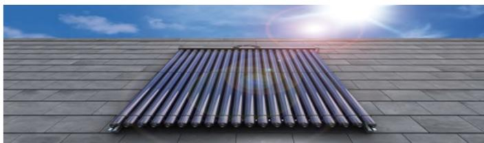
If correctly specified and installed, solar water heating can be very efficient. Good quality panels on a roof can supply 100% of hot water needs on sunny summer days to around 10% on a cloudy, winter's day, even in Scotland.
